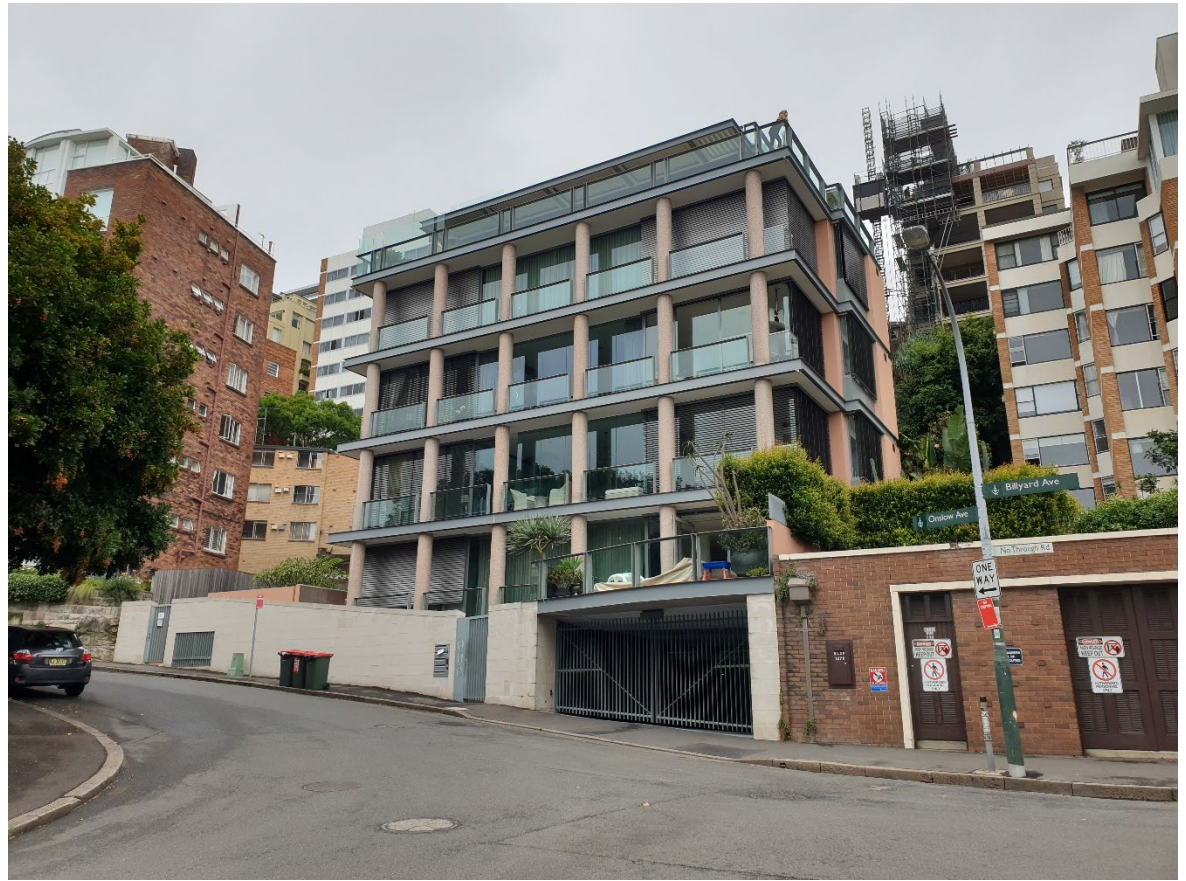
RFB at 1-3 Onslow Ave (left) & substation at 1A Onslow Ave (right)
